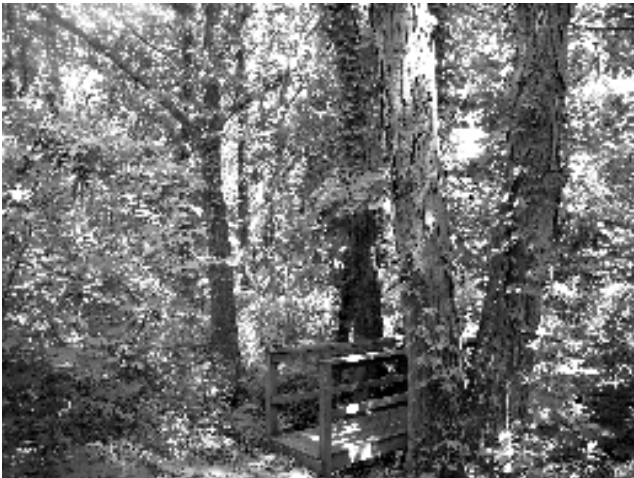
Another footbridge on the path.
